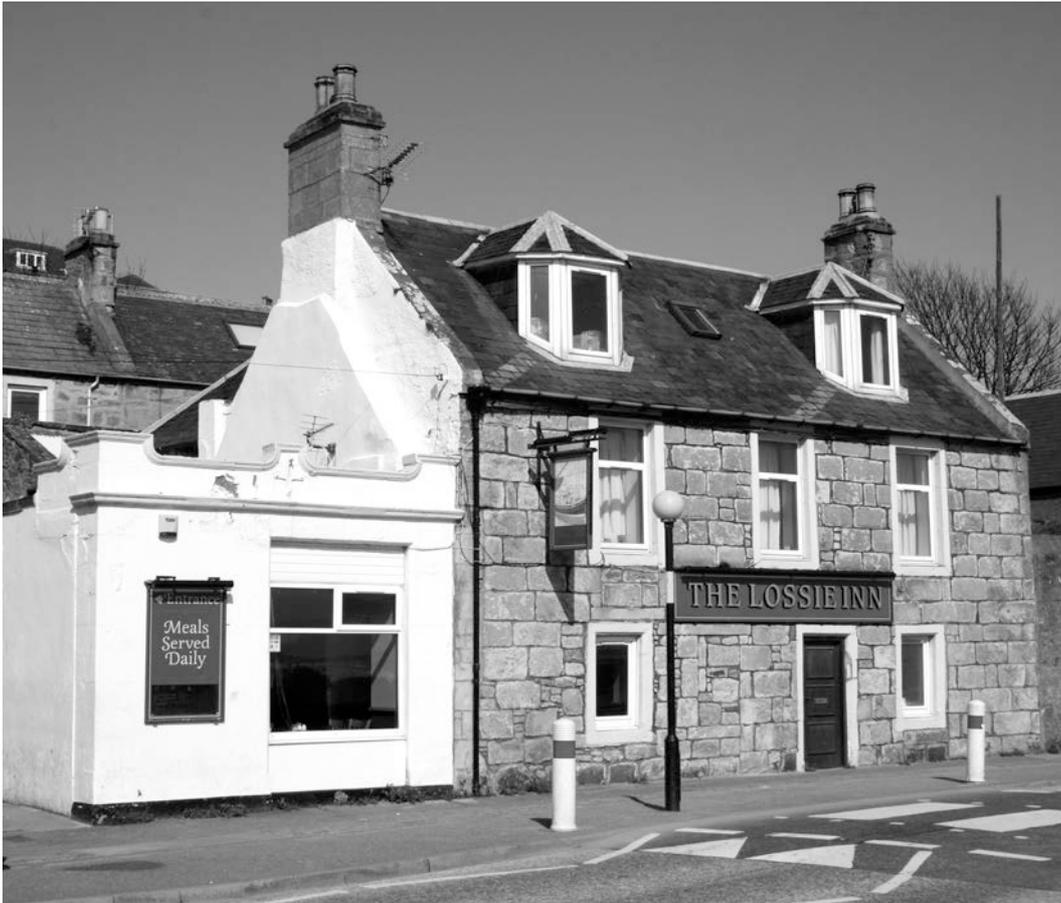
Figure 8. Comparable example from Lossiemouth, Scotland. Image shows use of local sandstone and five sided dormer windows
